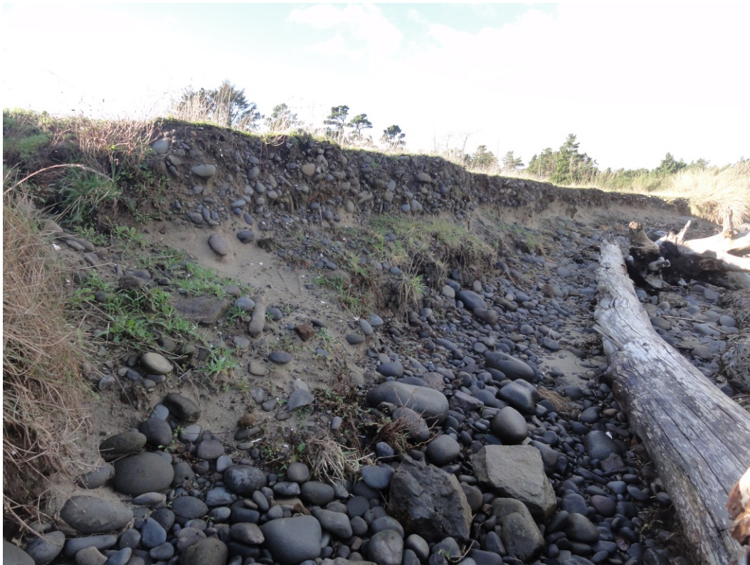
Figure 7. Cobble Fill in Profile at Helicopter Landing Site.
